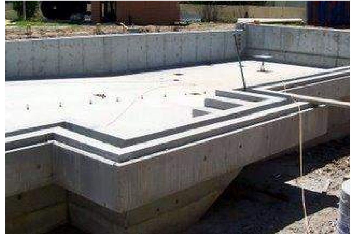
Figure 6.2: In-situ Reinforced Pool Tank Design at Grade
