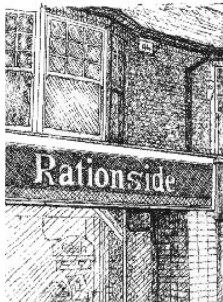
Figure 12 A shop front replacing a previous one that was related architecturally to the first floor facade. The deep, flat, box-fascia is over scaled for its location. The single paned shop window is framed in narrow flat strips of stainless steel and the flat sides of the pier on the right are clad in shiny glazed tiles. These features are not acceptable as they detract from the character of the building.
