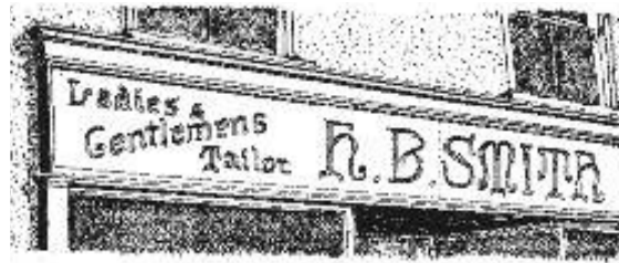
Figure 16 19th century signboard of slate with incised lettering, exposed from behind a modern shop signboard.
