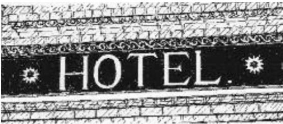
Figure 19 Sign painting direct to a rendered wall-face framed in moulded brick.
